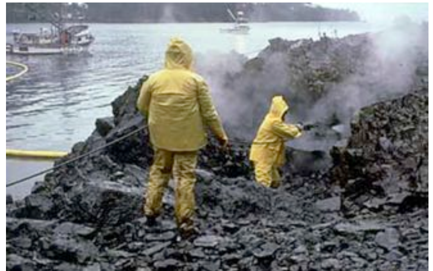
Workers using high-pressure, hot-water washing to clean an oiled shoreline near Prince William Sound after the Exxon Valdez spill.
